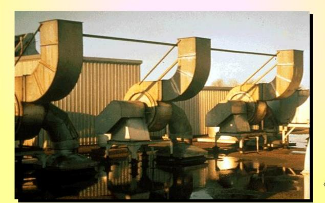
High loss inlet plenum without turning vanes: results in very high inlet pressure drop
