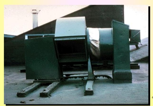
Short radius elbow close to inlet causes swirl & both inlet and outlet ducts result in high pressure losses
