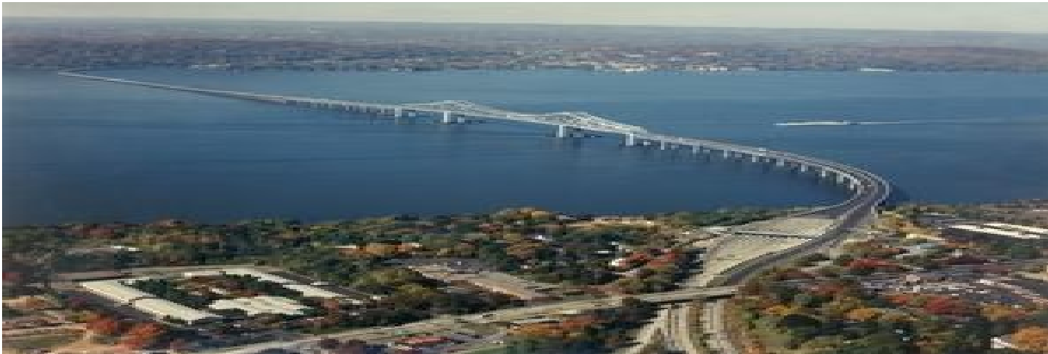
TAPPAN ZEE BRIDGE
